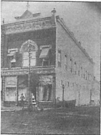
This is the original Bleckley Building and was built by Sylvester Bleckley. The next occupant of the building was Brown, Osborne and Company, a general merchandise store, then came Fleishman's Store. It was located on the east side of the square in what was known as Granite Row. It was the first building in Anderson to have an electric elevator powered by long-distance electricity from the pioneer hydro-electric plant at High Shoals. (Photo and information courtesy of Anderson Historian Beth Ann Klosky)
