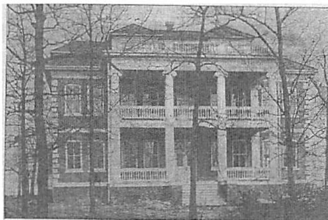
In 1904, Mrs. Jennie Gilmer was instrumental in building community support for a hospital to serve the residents of the Anderson area. The Anderson County Hospital Association was the result of her efforts. They raised $25,000 that was needed to construct the original two-story 25-bed hospital building that opened for operation in 1906. (Photo courtesy of Fred Whitten.)
